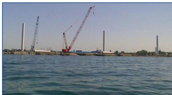
Construction of Steel Winds II
