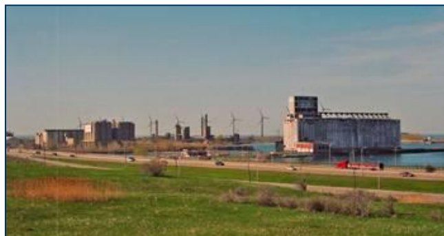
Steel Winds I – generating 20 MW
