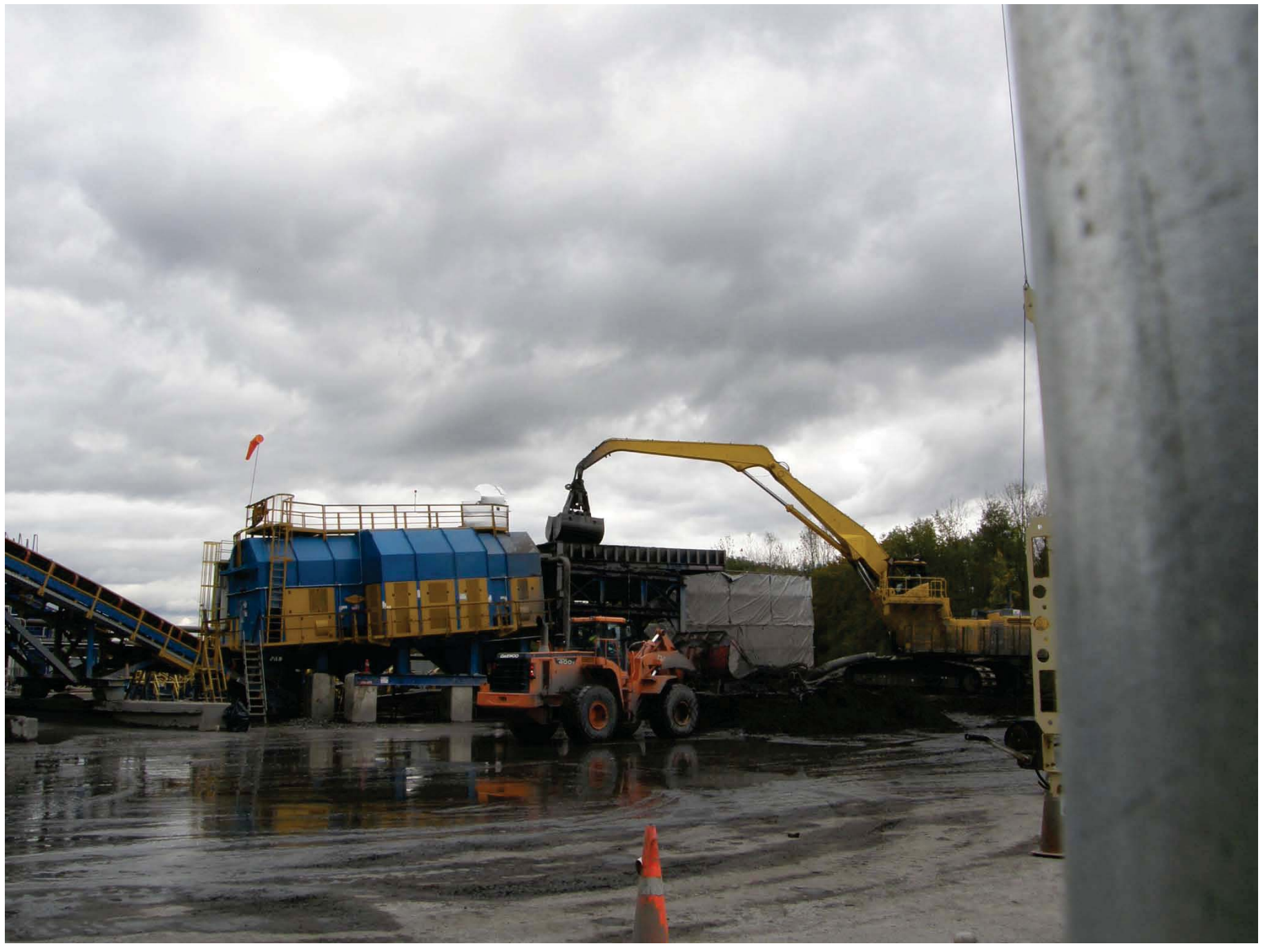
Komatsu Excavator Unloading Sediment Into Trommel Screen
