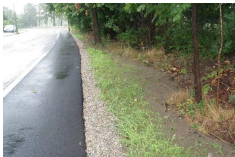
Infiltration trench (gravel) adjacent to a roadway.
