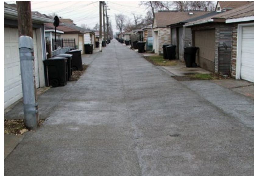
Permeable asphalt alley in Chicago, IL.
