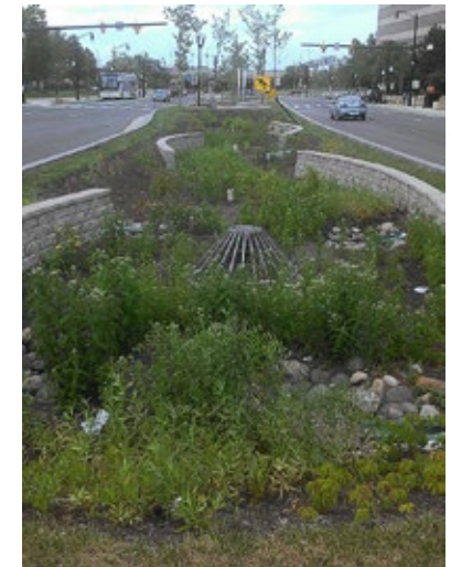
Figure 4-22. Beehive overflow grate prevents debris from entering the overflow structure in a roadside bioswale in Arlington, VA.
