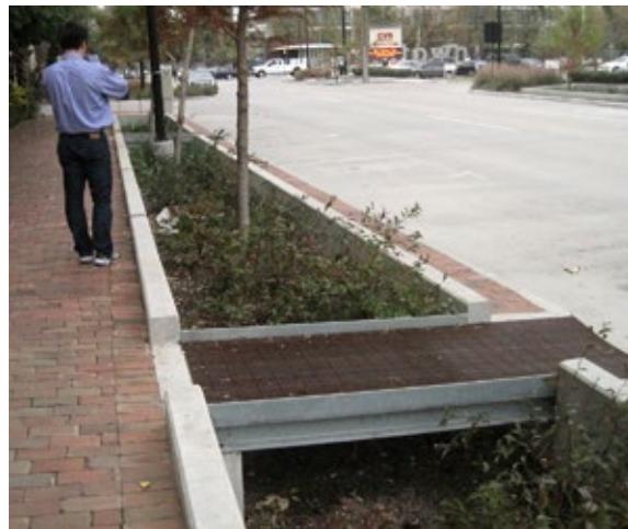
Figure 4-31. A grated walkway bridge allows pedestrians to access parked cars on Bagby Street in Houston, TX.
