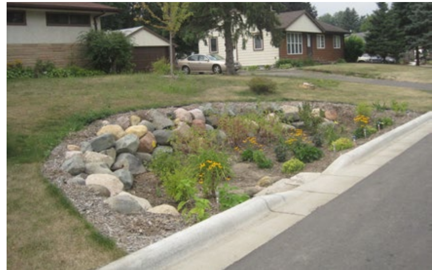
Road runoff drains through a curb cut and into this bioretention feature on a residential front yard in Maplewood, MN.
