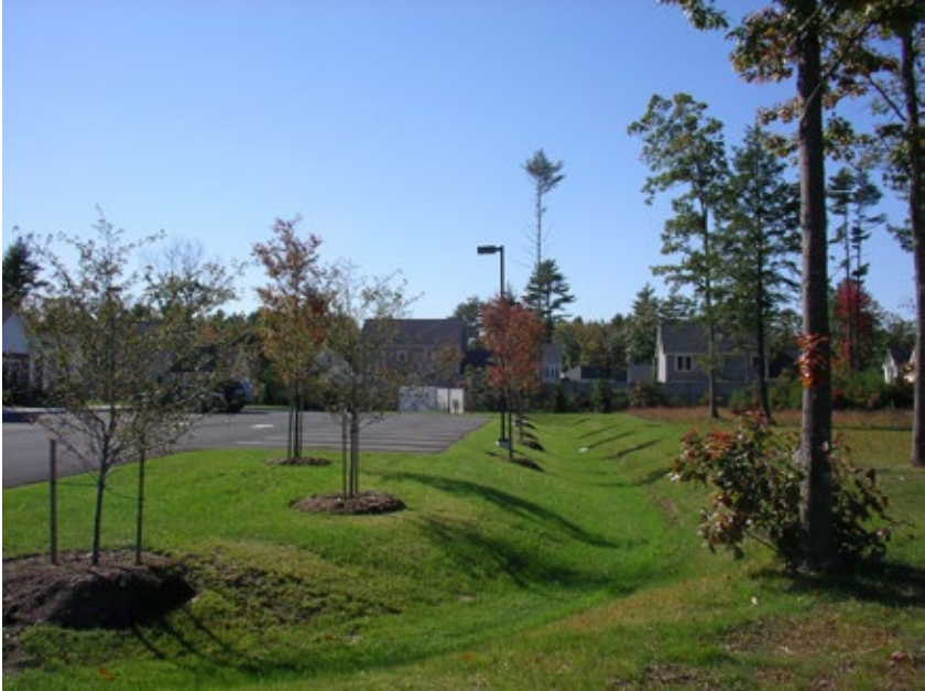
Grassed bioswale in New Hampshire.
