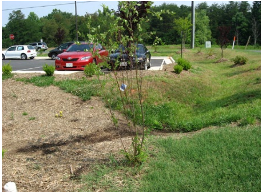
A pretreatment bioswale conveys and treats runoff from a parking lot and road in Stafford, VA.
