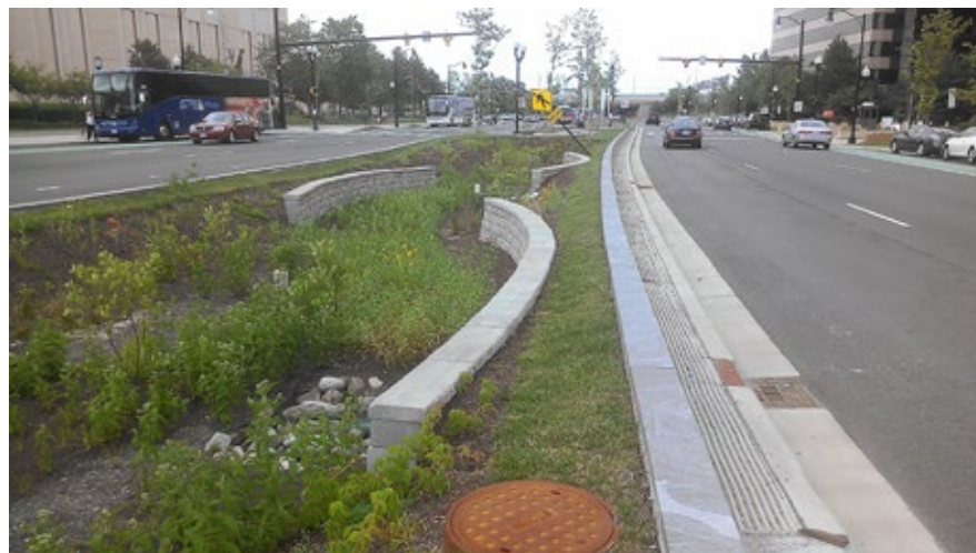
Medians with rain gardens manage stormwater runoff from the street collected via stormwater inlets connected to subsurface pipes in Arlington, VA.
