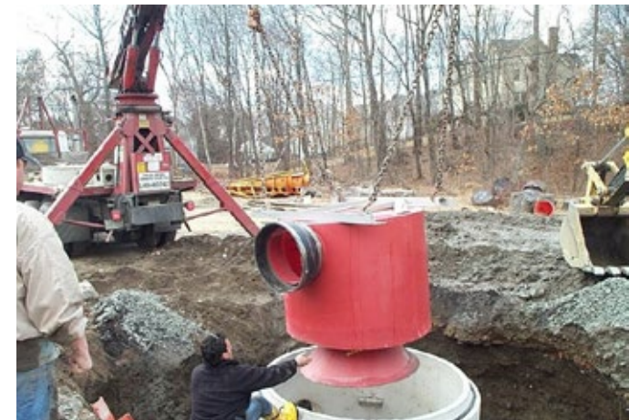
Vortex separator being installed.
