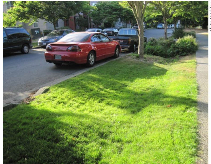
Grass swale serves as pretreatment for a bioretention area in the High Point neighborhood in Seattle, WA.
