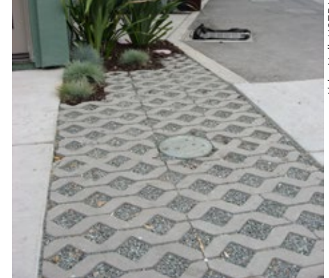
Concrete grid pavers in Emeryville, CA.
