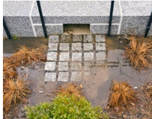
Figure 4-15. Concrete paver splashpad dissipates energy from stormwater entering from a trench in Washington, DC.
