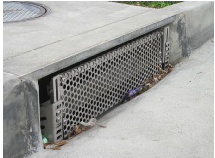
A curb inlet cover allow runoff to enter a catch basin but prevents inflow of trash.
