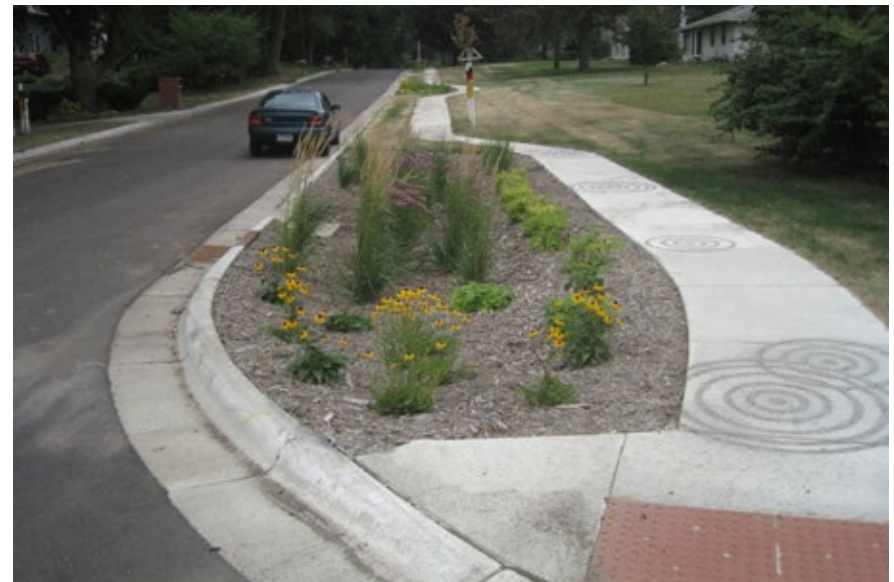
Stormwater curb extension installed with a sidewalk project in Maplewood, MN.
