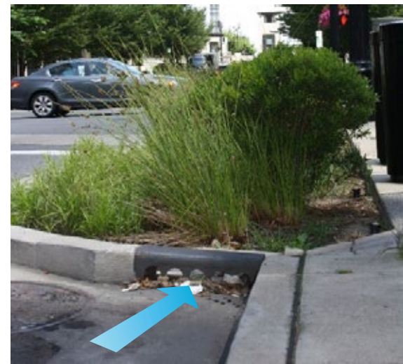
Figure 4-8. A grated inlet prevents large floatable trash from entering practice along Deaderick Street in Nashville, TN.
