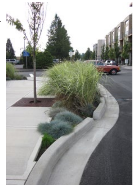
Mature grasses and a tree pit treat stormwater in a curb extension in Gresham, OR.
