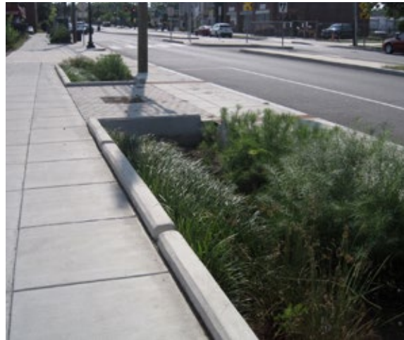
Figure 4-33. A raised curb with inlets defines the edges of a sidewalk stormwater planter in Washington, DC.
