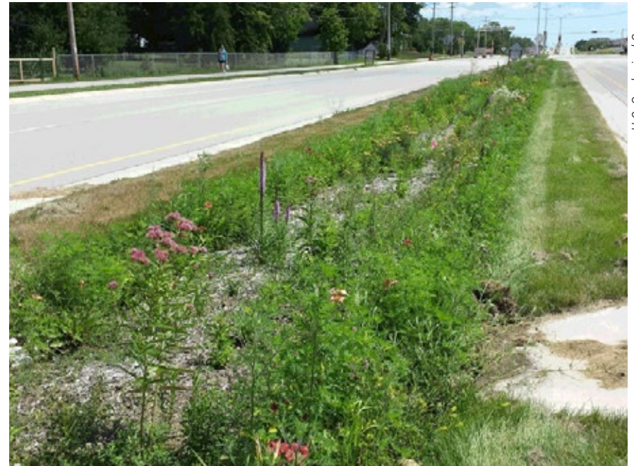
A bioretention area located in the median of an arterial road captures runoff in the Great Lakes region.
