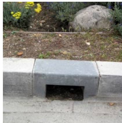
This undersized curb cut is easily clogged by mulch and other debris.
