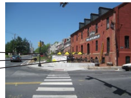
Figure 2-16. A roadway was reconfigured to replace a turn lane with green infrastructure practices in Lancaster, PA.
