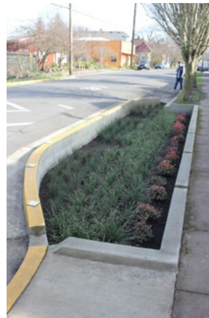
Densely planted low-growing grasses fill a stormwater curb extension in Portland, OR.
