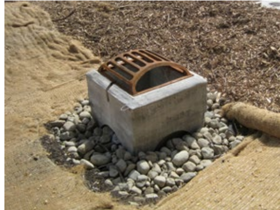
The large-spaced grate on this overflow drain will not prevent floatables and debris from entering.
