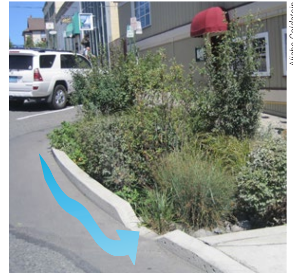
Figure 4-6. A curb cut with 45-degree chamfered edges conveys stormwater into a roadside rain garden in Friday Harbor, San Juan Island, WA.
