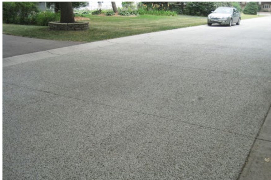
Pervious concrete pavement on a low-speed residential roadway in Shoreview, MN.
