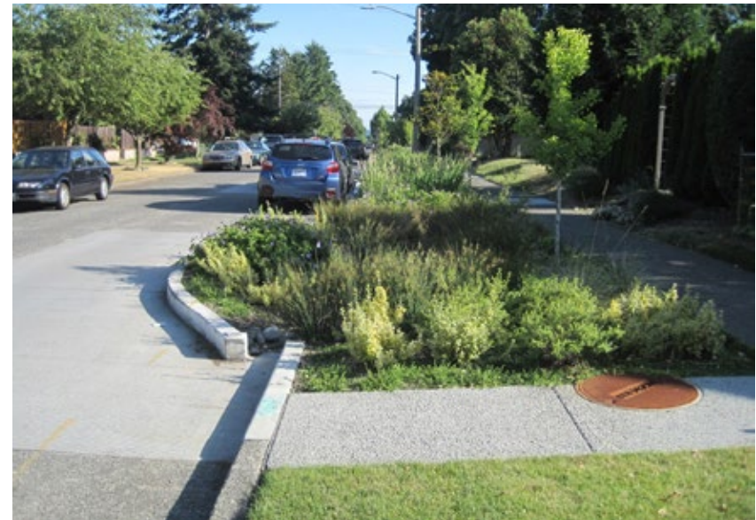
Parking impacts minimized by using a mid-street stormwater curb extension in the Barton Creek neighborhood, Seattle, WA.
