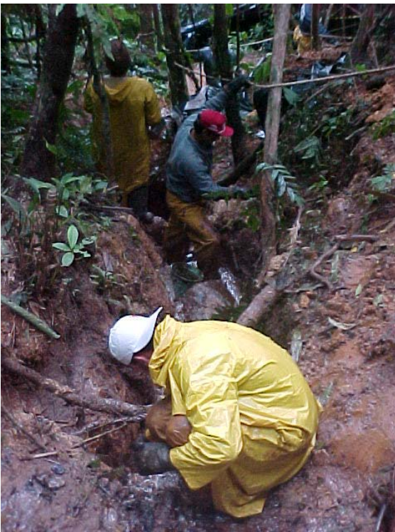
Fig. 17 – Workers cleaning one of the “tracks”.
