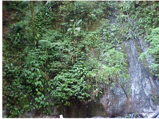
Fig. 10 – Partial view of the rock wall.
