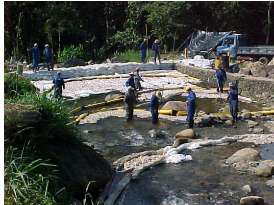
Fig. 24 – Upstream view of the dam.
