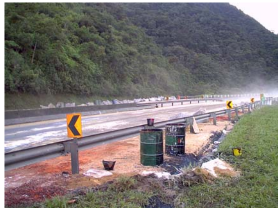
Fig. 6 – Road cleaning and decontamination.
