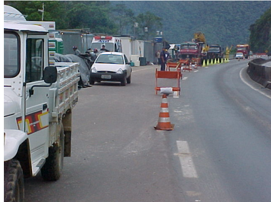
Fig. 14 – Operational base on the roadside.
