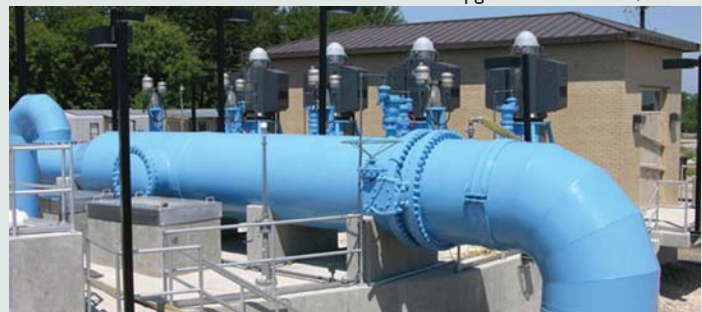
ARRA-funded infrastructure upgrades in Amarillo, Texas
