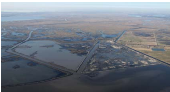
Aerial View of mid-construction of Marsh Creation/ Marsh Nourishment Project Area
