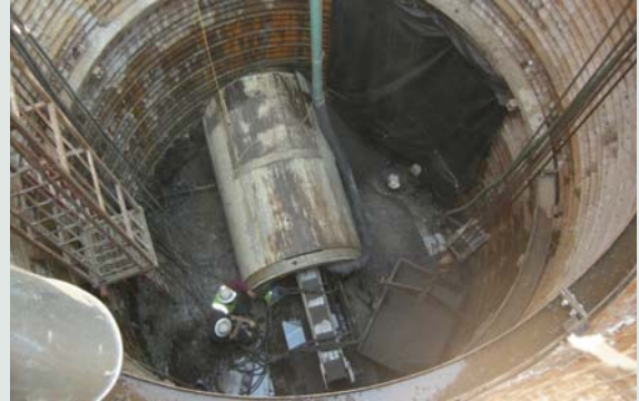
ARRA funding at work in Batesville, Arkansas
