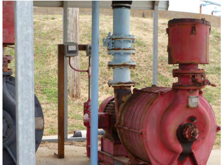
Old pumps slated for replacement
