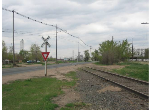
Site Identified for a new light rail station by the Commerce City Planning Department.
