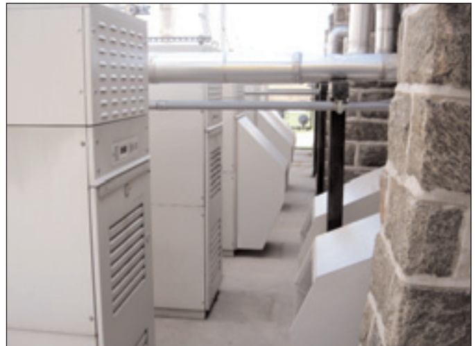
Microturbine Installation at Masonic Homes.
