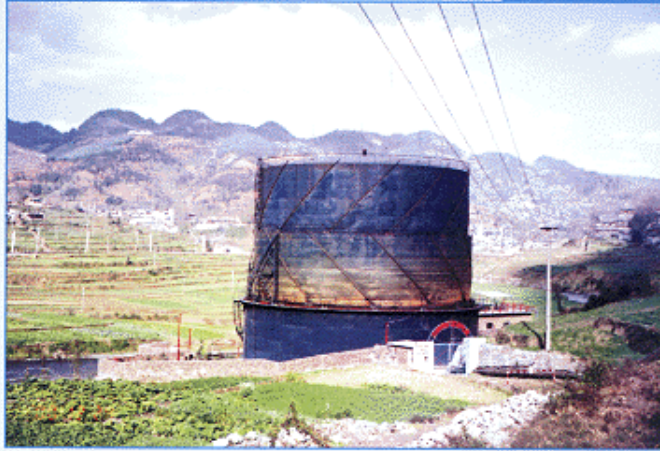
Two gas holders have been built in Panjiang mining area, with total storage capacity of 20,000 m 3 .
