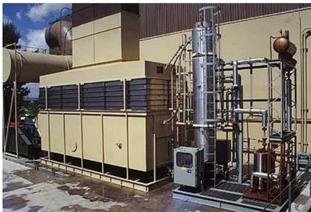
Figure 6. Environmental C & C's Fluidized Bed Concentrator
