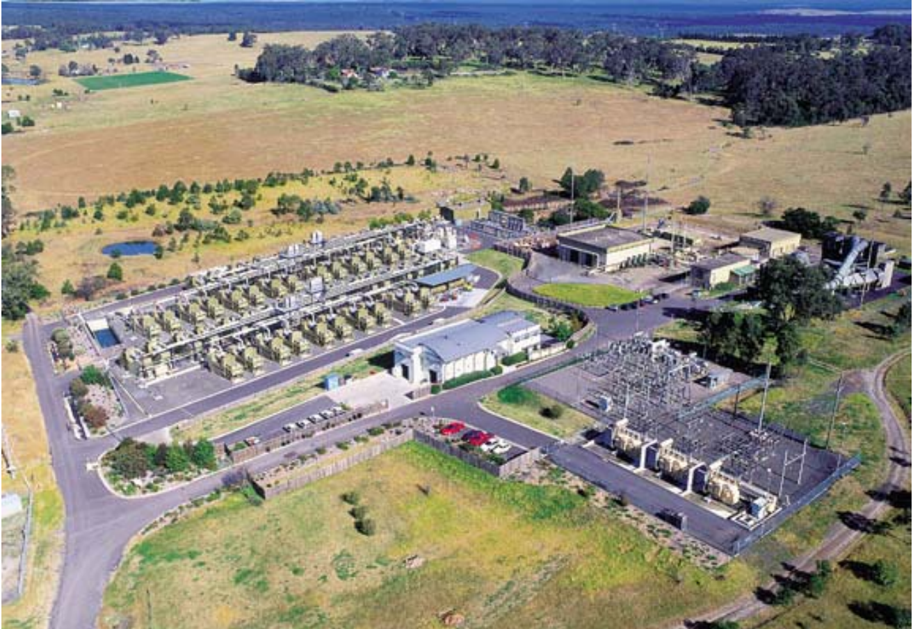
Appin Power Plant, New South Wales, uses VAM as combustion air in its IC engines (Photo courtesy of Energy Developments Limited)
