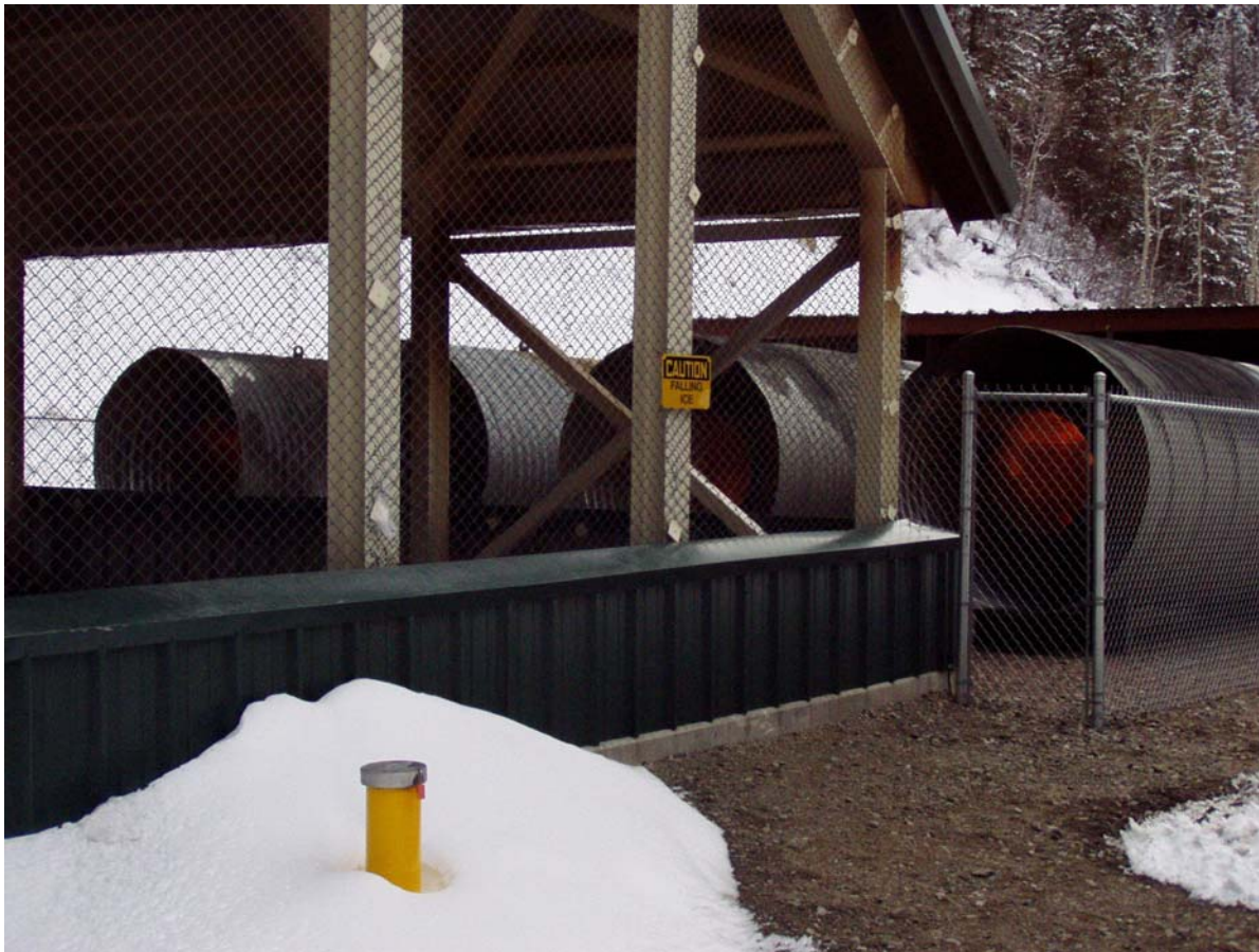
Coal mine methane-fueled heaters at a mine in the Rocky Mountains (Photo courtesy of Raven Ridge Resources, Incorporated)
