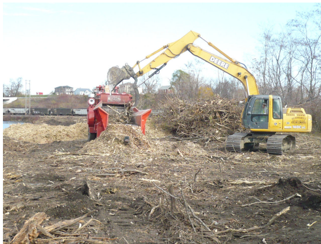
Crews prepare the peninsula at 5 ½ slip for habitat restoration work.
