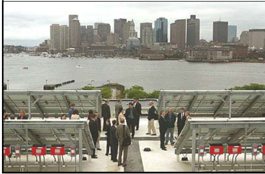
Maverick Gardens, Boston Housing Authority, 33 kW Photo Voltaic System
