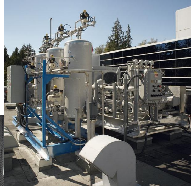
Test Gas Recirculation
