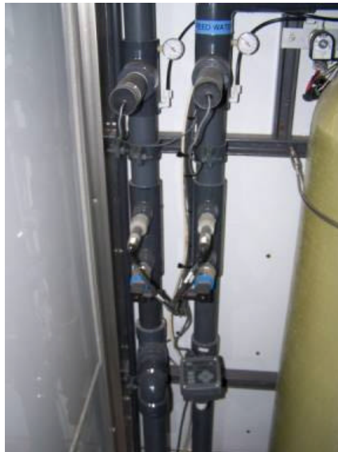
Photograph 5: Inline pressure, flow, pH and conductivity meters.
