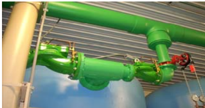
A drinking water project in North Manchester, Indiana. (EPA OIG)
