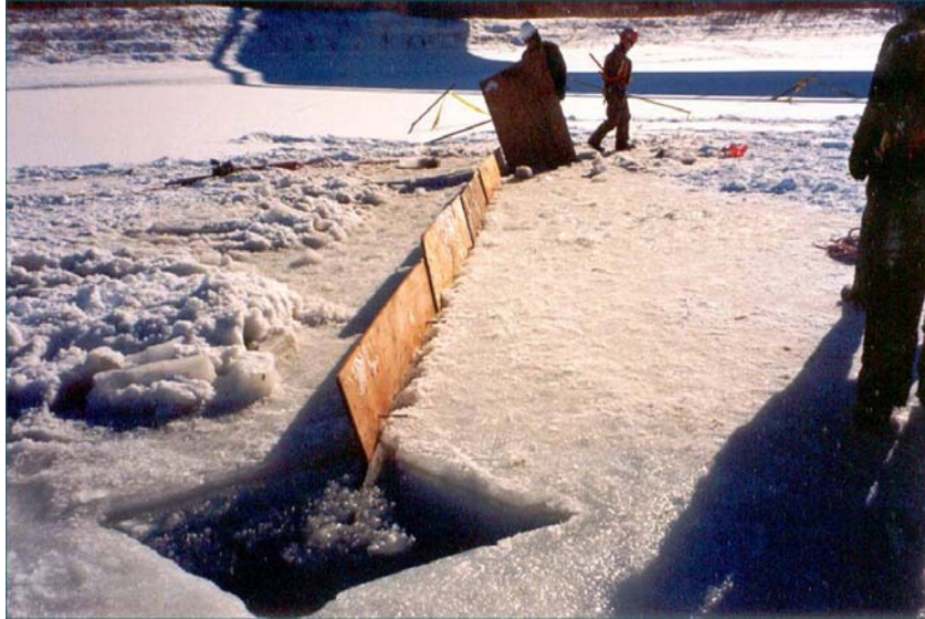
Figure 3. Diversionary Plywood Barrier Method
