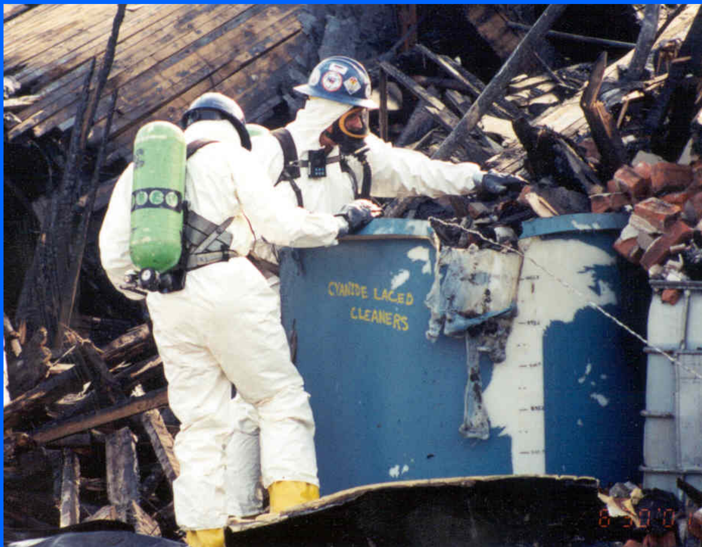
Chemical Plating Facility Fire – Detroit, MI - 2001
