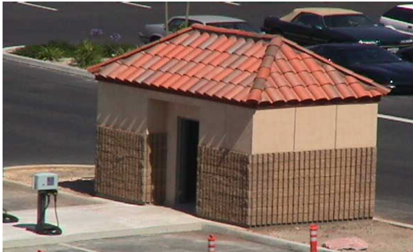
Figure 4 SUVMS Communications Equipment Enclosure
