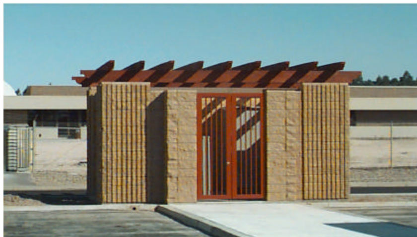
Figure 3 SUVMS Electrical Equipment Enclosure
