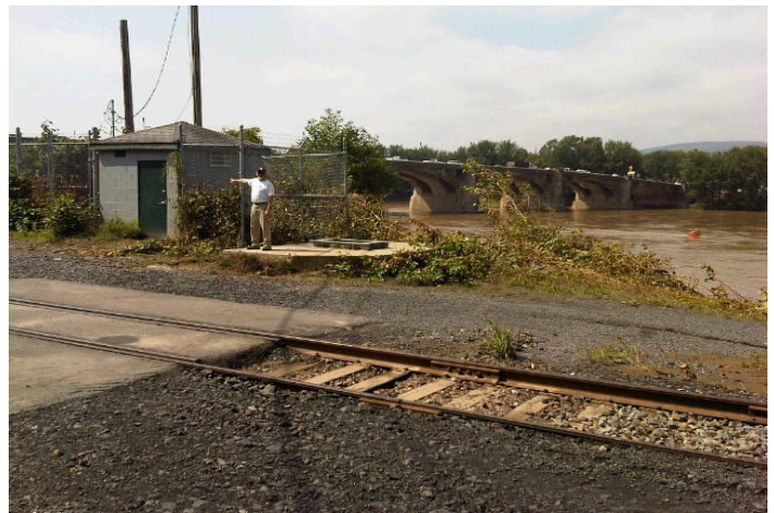
EPA On-Scene Coordinator Inspects the Site
