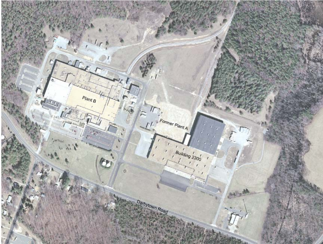
Figure 1. Pfizer Facility and Surrounding Area. (September 2007)
