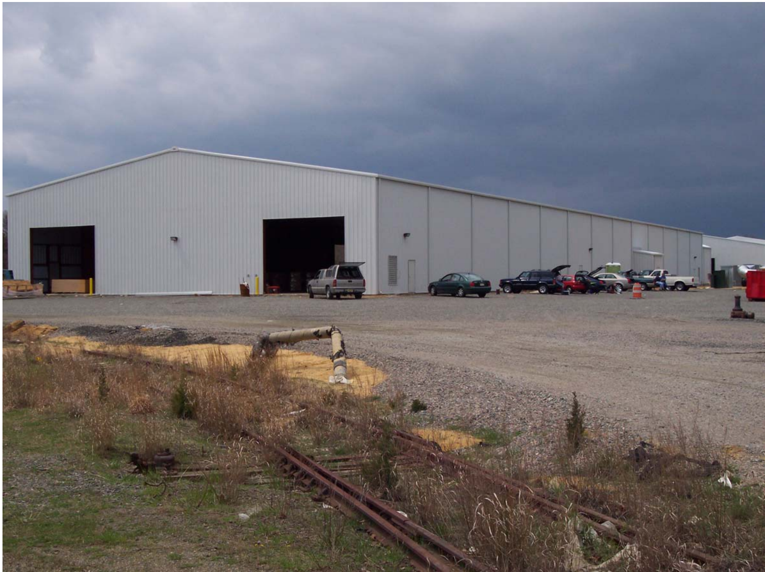
The soil storage building, which is 100 feet wide, 344 feet long and 20 feet high, will hold approximately 7000 cubic yards of contaminated soil from several different source areas.
