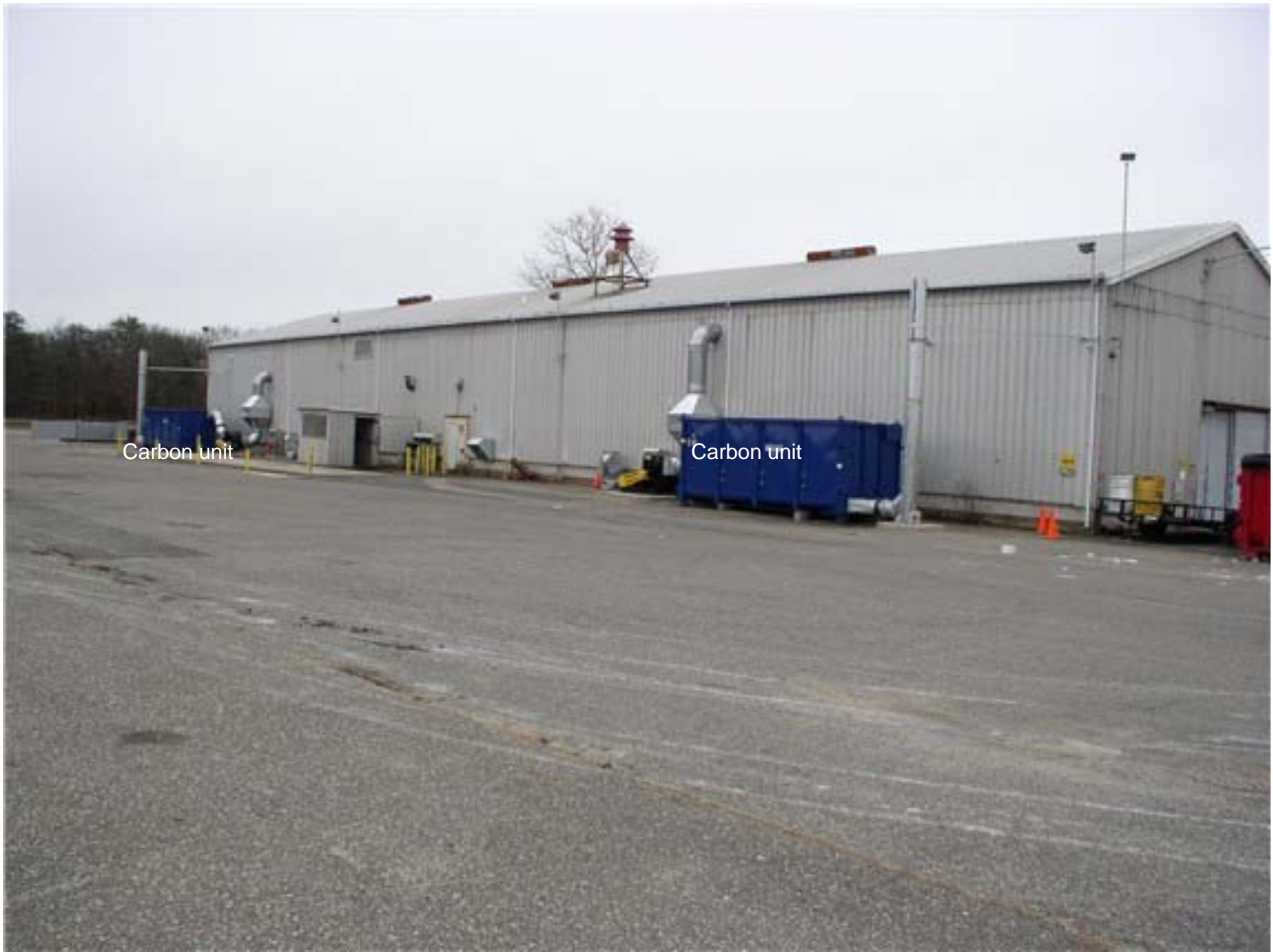
Air from the Drum Handling Building is treated in two carbon units before being released to the atmosphere.
