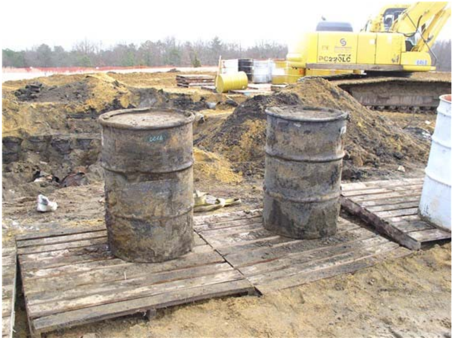
Drum removal began on December 9, 2003.
