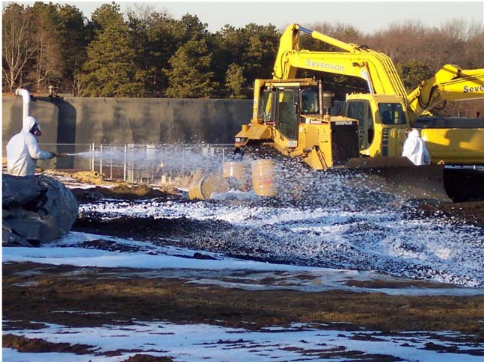
The excavation can be foamed to reduce emissions and odors.
