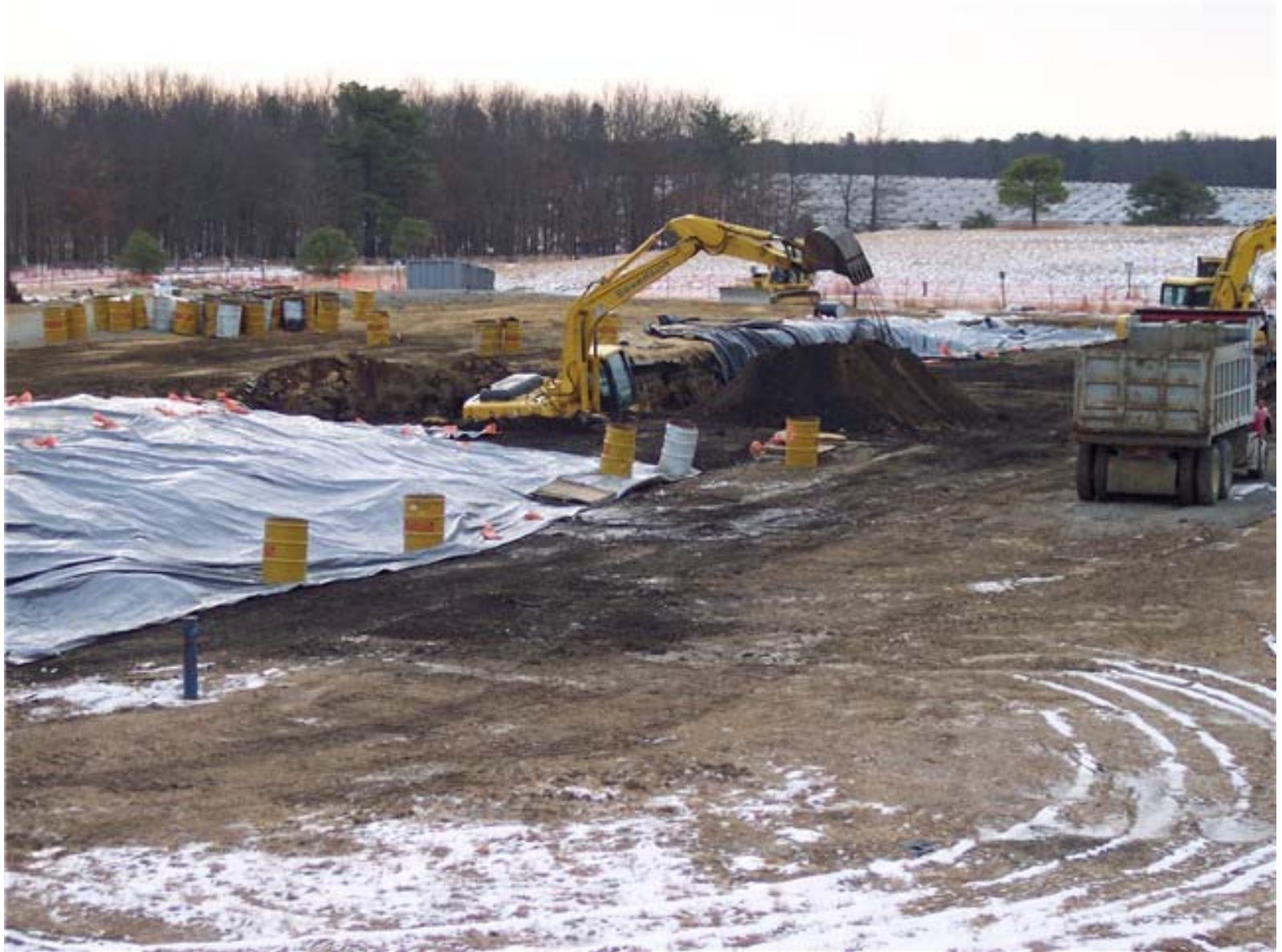
Soil from around drums is stockpiled and will be treated on Site in the bioremediation facility.
