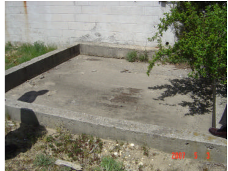
Area Q (1,750 Gallon Caustic Sludge Storage Tank), View to the Northwest
