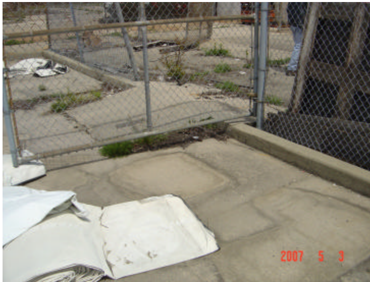
Area J, View to the North
