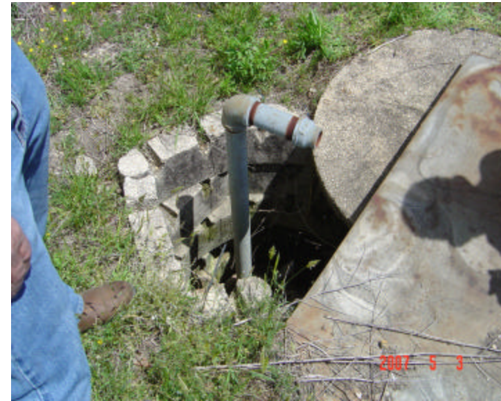
Former Plant Production Well
