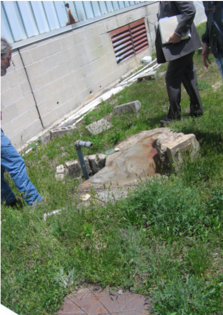
Former Plant Production Well, View to the Northeast
