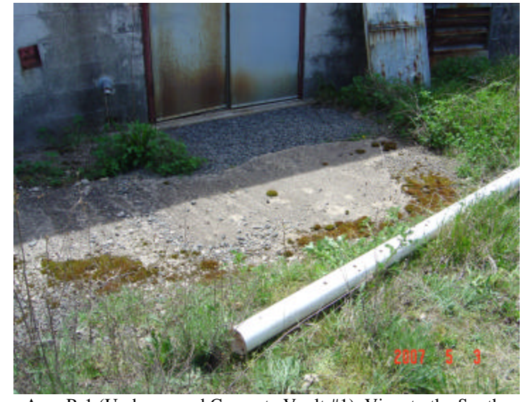
Area P-1 (Underground Concrete Vault #1), View to the Southwest
