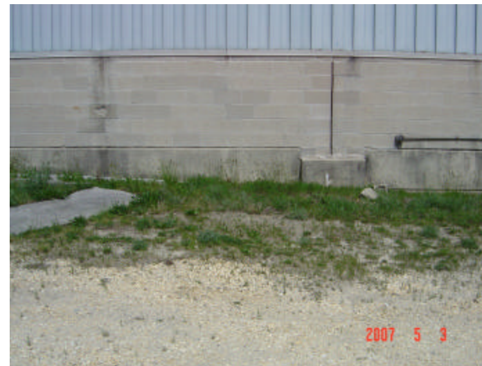
Area I (Former Empty Chromate Storage Area), View to the North
