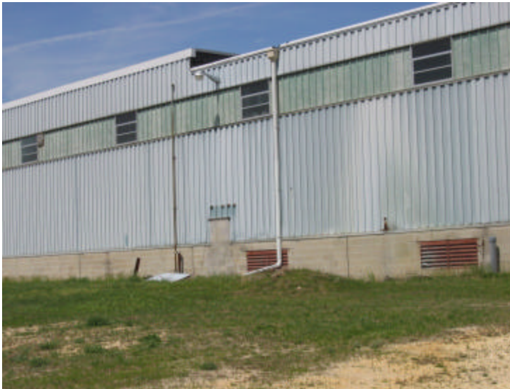
Production Building & Maintenance Shop, View to the Northwest
