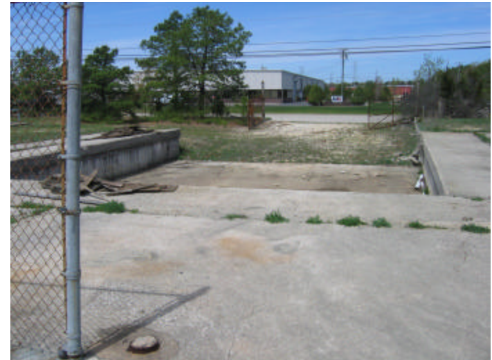
Area K 9 (Concrete Storage Pad), View to the North
