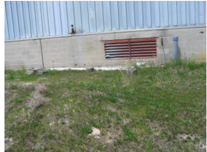
Area H (Former Compressor Blowdown Area), View to the Northwest
