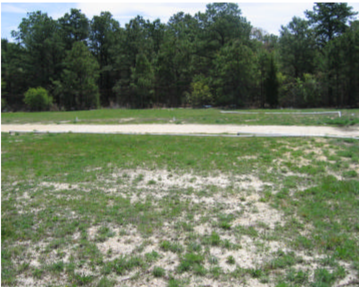
Soil Venting/Sparging System - Piping
