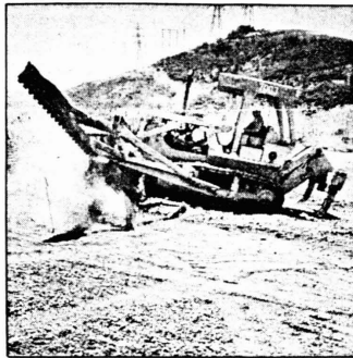
Fred Moeller guides his 25-ton bulldozer over a mound.
