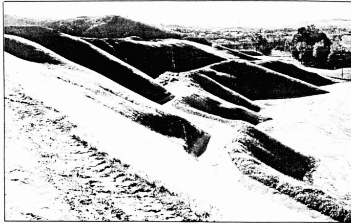
Landform grading sculpts the hillside of Talega project into new shapes in technique created by Horst Schor.
