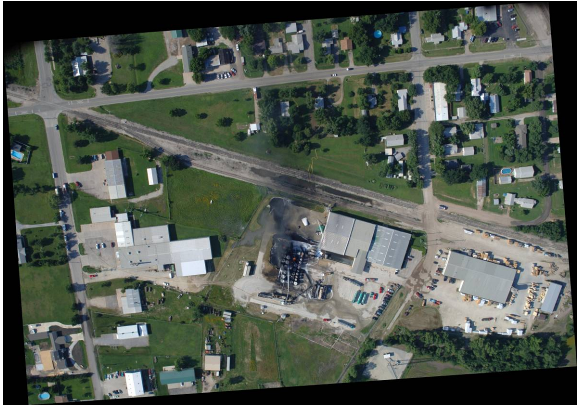
Figure 1. Aerial Image Data Pass 4, Sortie II, Barton Solvents, Valley Center, Kansas
