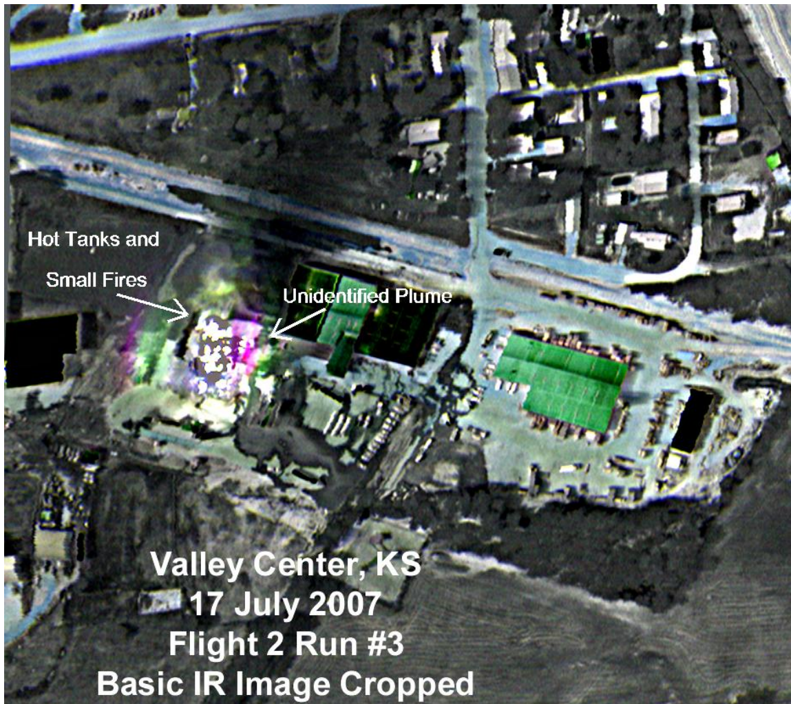
Figure 3. IR image Run 3 – Sortie II, Barton Solvents, Valley Center, Kansas
