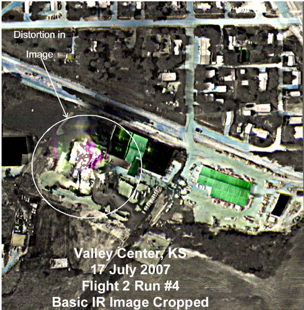
Figure 4. IR image Run 4 – Sortie II, Barton Solvents, Valley Center, Kansas
