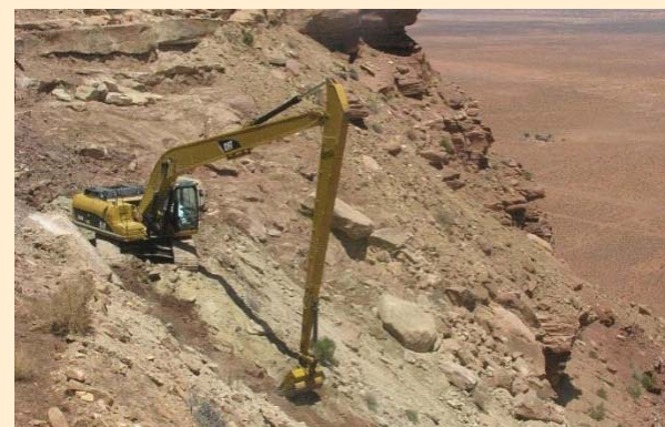
Large scale cleanup at Skyline Mine
