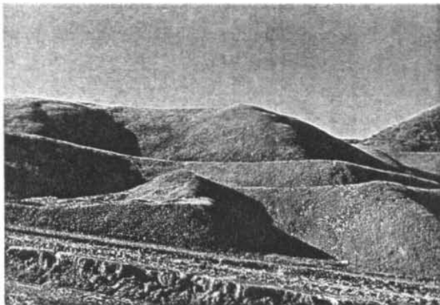
FRESHLY GRADED landform slopes show ridges, swales and pyramid shapes.
