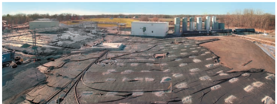
Piping for the SBPA ISVE installed above the clay and geotextile layers.
