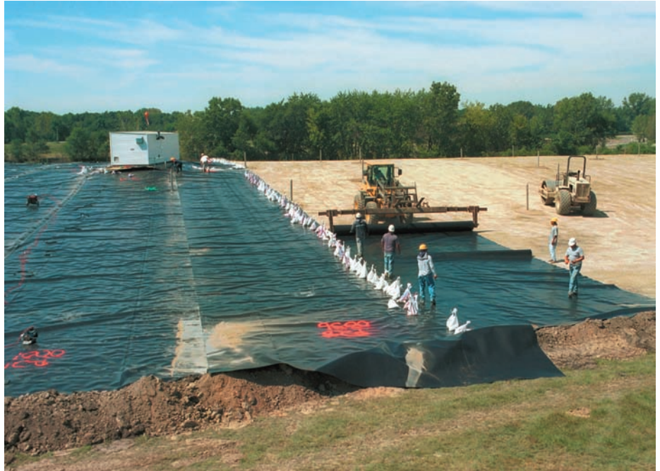
Flexible liner being installed over sections in the off-site area. Rolls of the liner materials 23-feet wide and 500-feet long were unrolled using a special forklift attachment.
