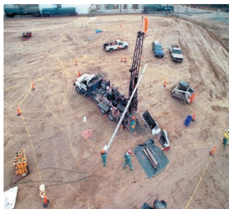
A DPE well being installed in the SBPA ISVE system.
