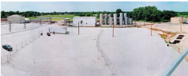
SBPA ISVE Area after placement and compaction of the gravel layer.
