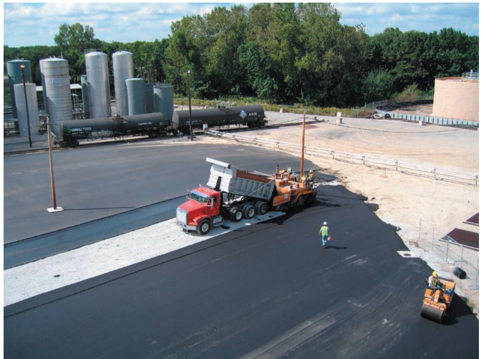
Placement of asphalt cover to the SPBA ISVE Area.
