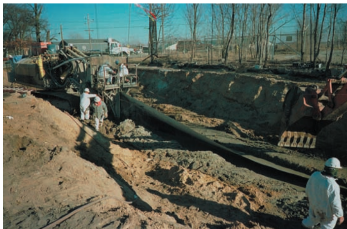
Trencher at the south side of the site installing the Perimeter Barrier Wall. The HDPE liner is shown stretched out behind the trencher, with the bentonite slurry along both sides of the liner.
