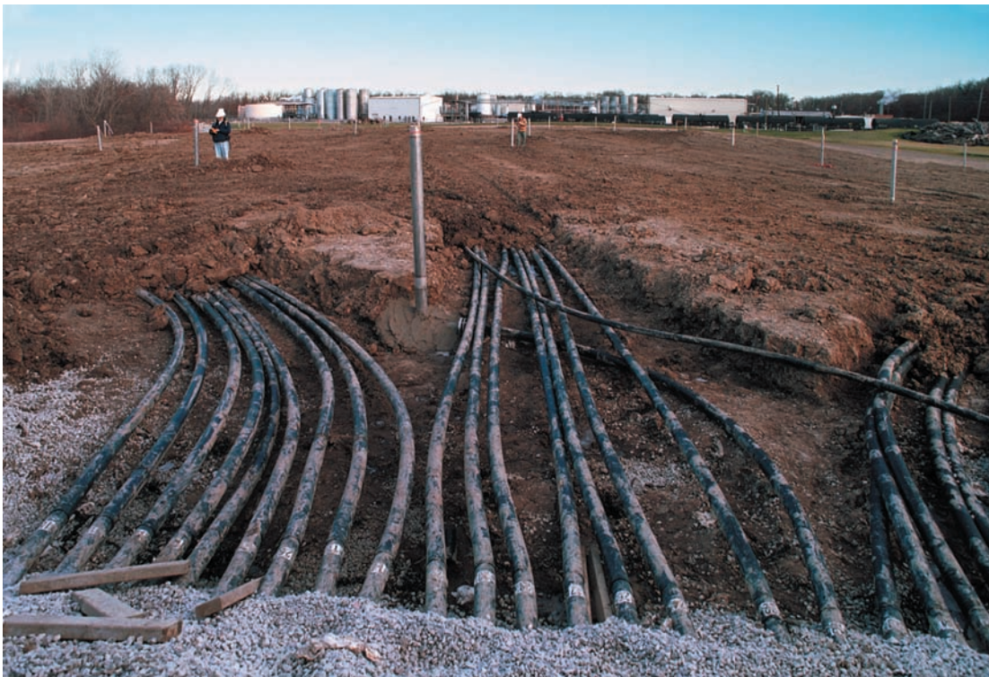
The completed ISVE piping for wells north of the blower shed. At the time of this photograph, the ISVE well and piping in the foreground have yet to be backfilled. A bentonite plug is visible at the base of the nearest well in the center of the photo. The plug provides an additional seal for the connection between well and piping. The smaller diameter pipe crossing over the others is piping associated with one of three air sparge points.
