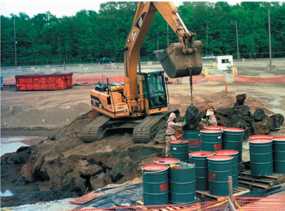
Intact drums in Area A being placed in over-pack containers. After all the drums had been removed the excavation was dewatered, filled with clean soil, and then compacted.
