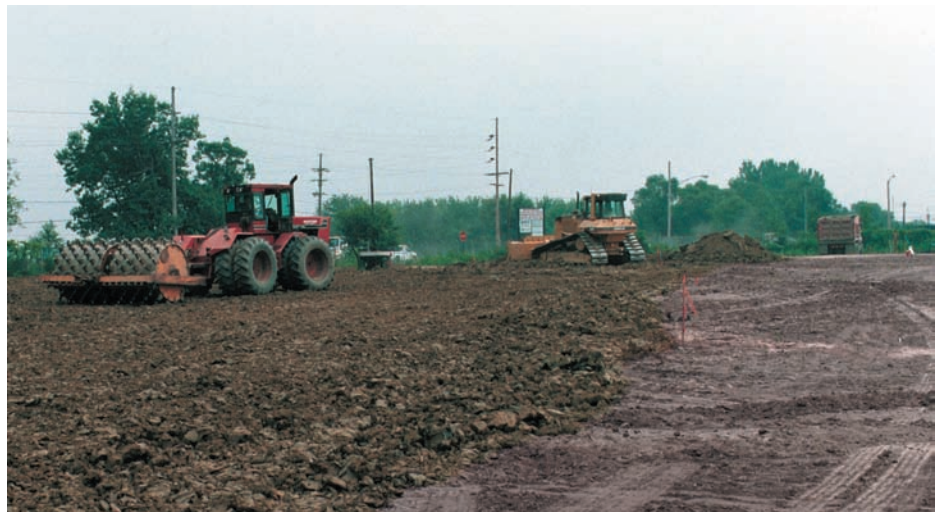
Construction of the Off-Site Area interim cover. A continual stream of dump trucks brought the loads of clean clay into the site. A bulldozer spread the clay in six-inch lifts, which were then compacted by repeated passes
