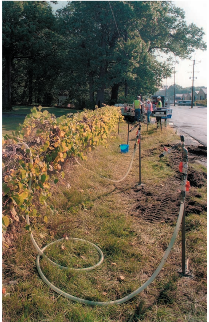
Portion of the treatment array with injection points located along Colfax Avenue during Phase I of the chemical oxidation application.
