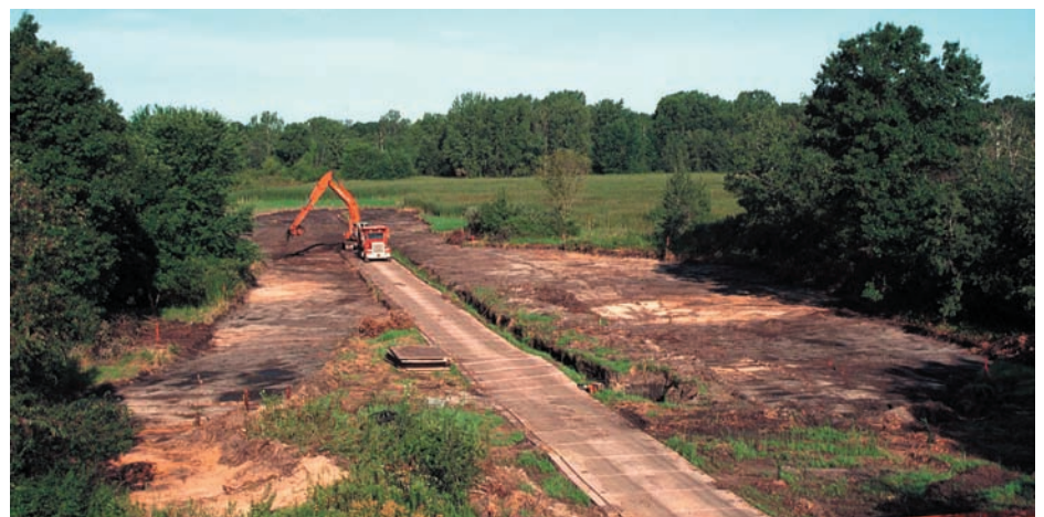
PCB-impacted sediment being removed from the wetland area in August 2001.
