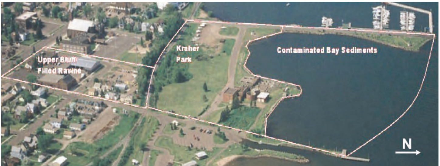
Aerial photo shows the Ashland Lakefront site. The “Upper Bluff/Filled Ravine includes the location of the former manufactured gas facility that created much of the pollution on the site.
