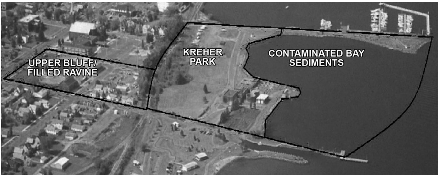
Aerial photo shows the Ashland/NSP Lakefront site. The Upper Bluff/Filled Ravine includes the location of the former manufactured gas facility that created much of the pollution on the site.
