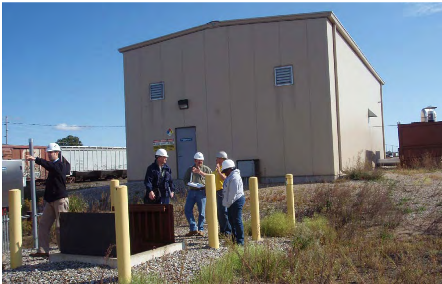
Rail Yard Treatment Plant
