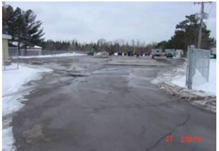
This photo shows the cleared site after the building and all waste was removed.
