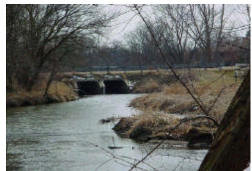
Kress Creek from the outfall.
