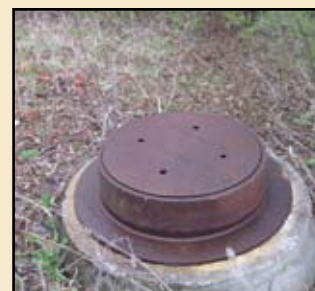
Wells similar to this have been installed to monitor water quality.
