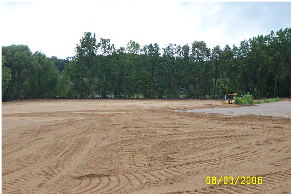
Rockwell site looking northeast. 8/4/06
