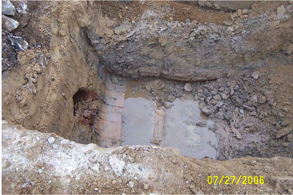
Remnants of clay sewer line near MH-11. 7/27/06
