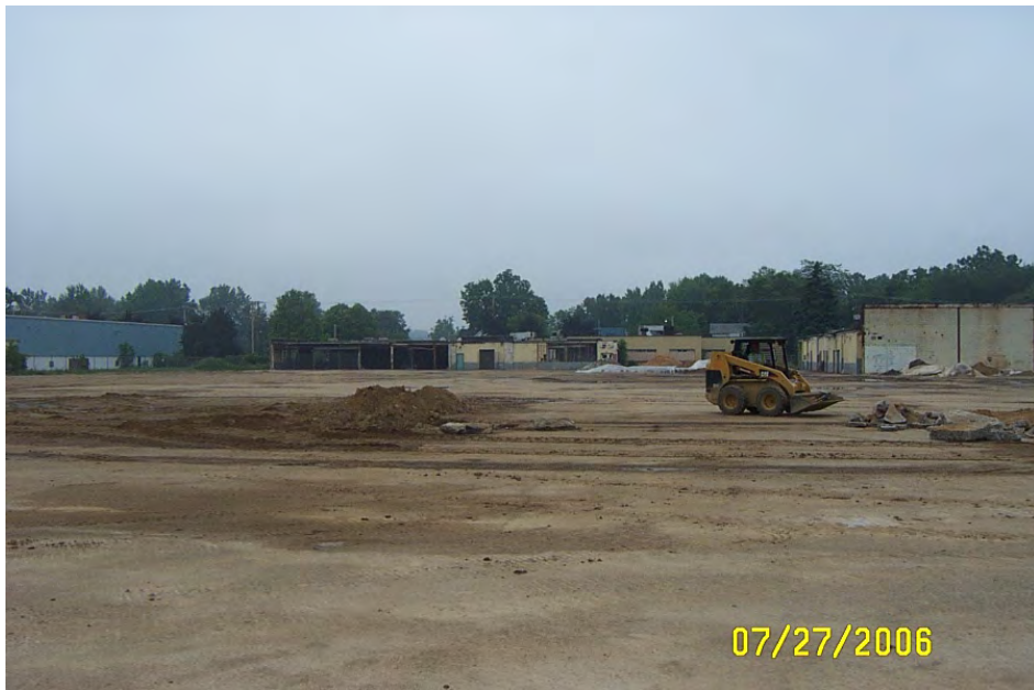
Sewer line excavation looking south. 7/27/06
