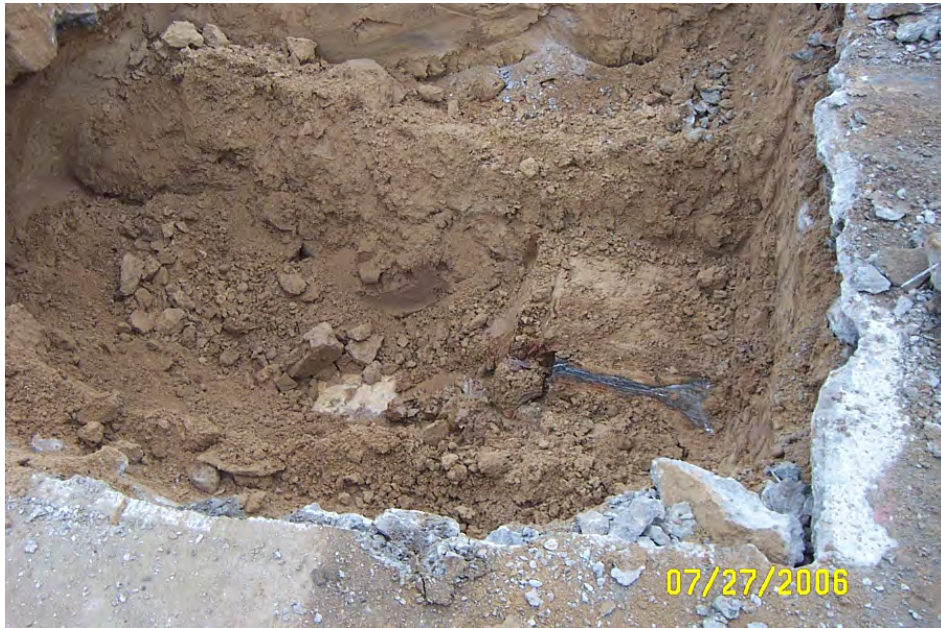
Remnants of clay sewer line near MH-11. 7/27/06
