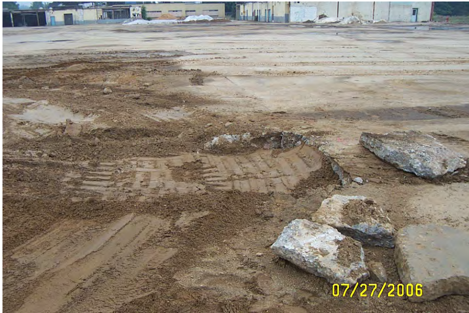
Sewer line excavation looking south. 7/27/06
