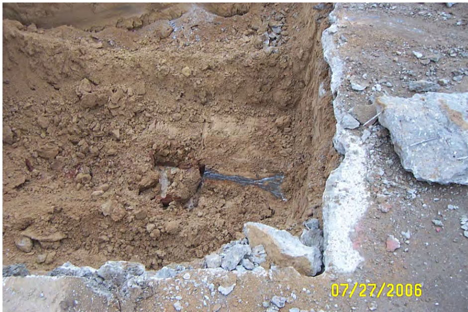
Remnants of clay sewer line near MH-11. 7/27/06
