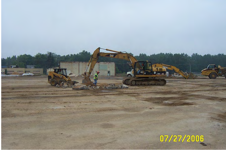
Sewer line excavation looking south. 7/27/06
