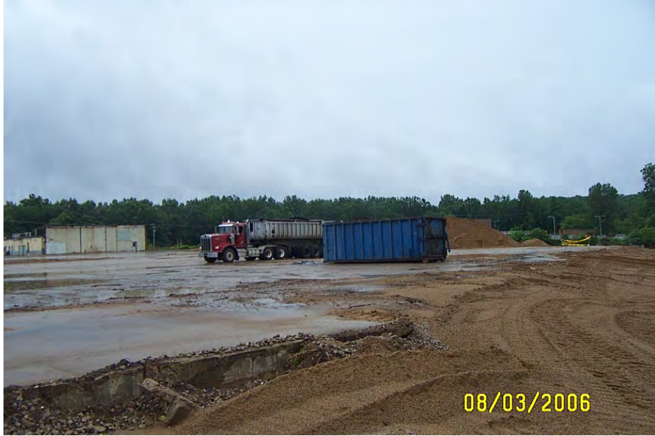
Trucks dumping backfill sand for grading and finishing purposes. 8/4/06
