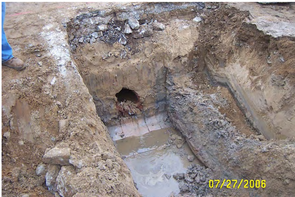
Remnants of clay sewer line near MH-11. 7/27/06
