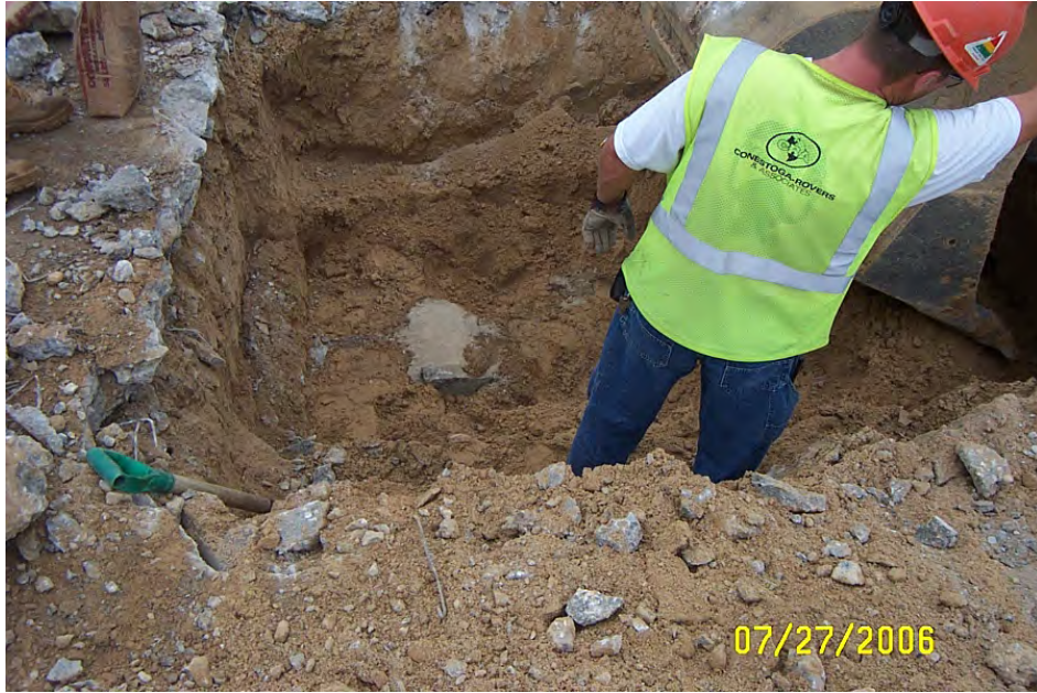
Remnants of clay sewer line near MH-11. 7/27/06
