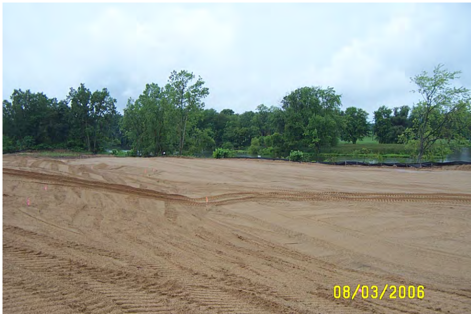
Rockwell site looking northwest. 8/4/06
