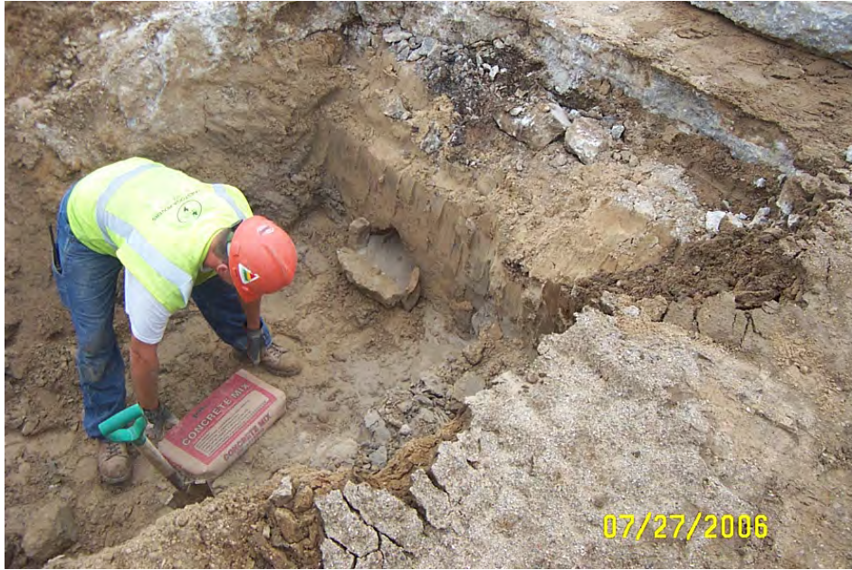
Cementing remnants of clay sewer line near MH-11. 7/27/06
