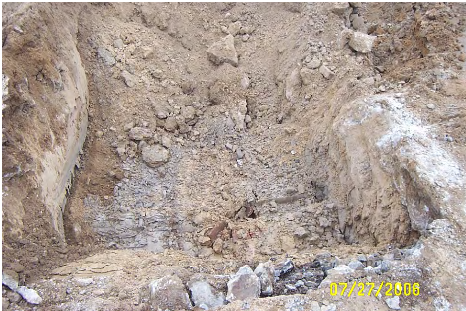
Remnants of clay sewer line near MH-11. 7/27/06
