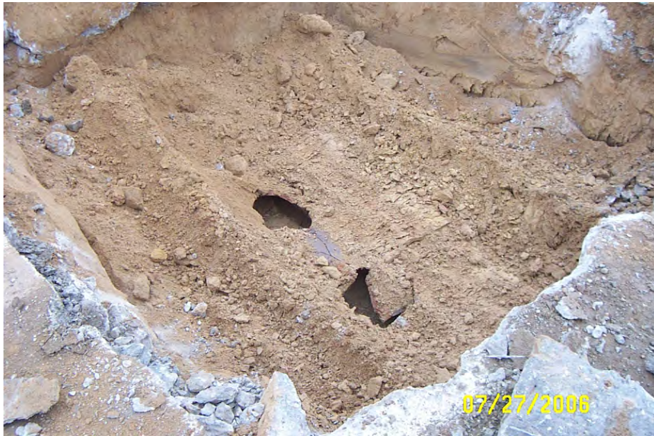
Remnants of clay sewer line near MH-11. 7/27/06
