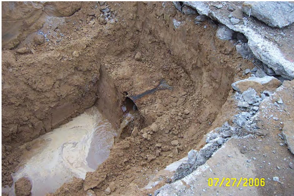
Remnants of clay sewer line near MH-11. 7/27/06
