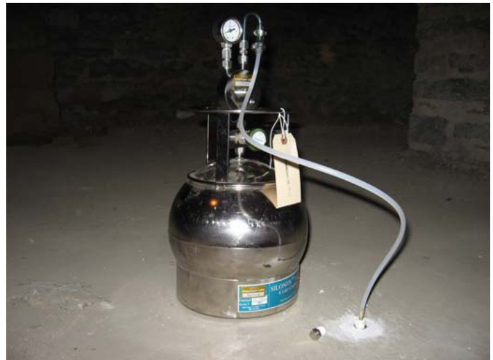
In this example of “sub-slab” sampling, tubing is run from underneath a basement floor to a “Summa” canister to test for hazardous vapors trapped in the soil.
