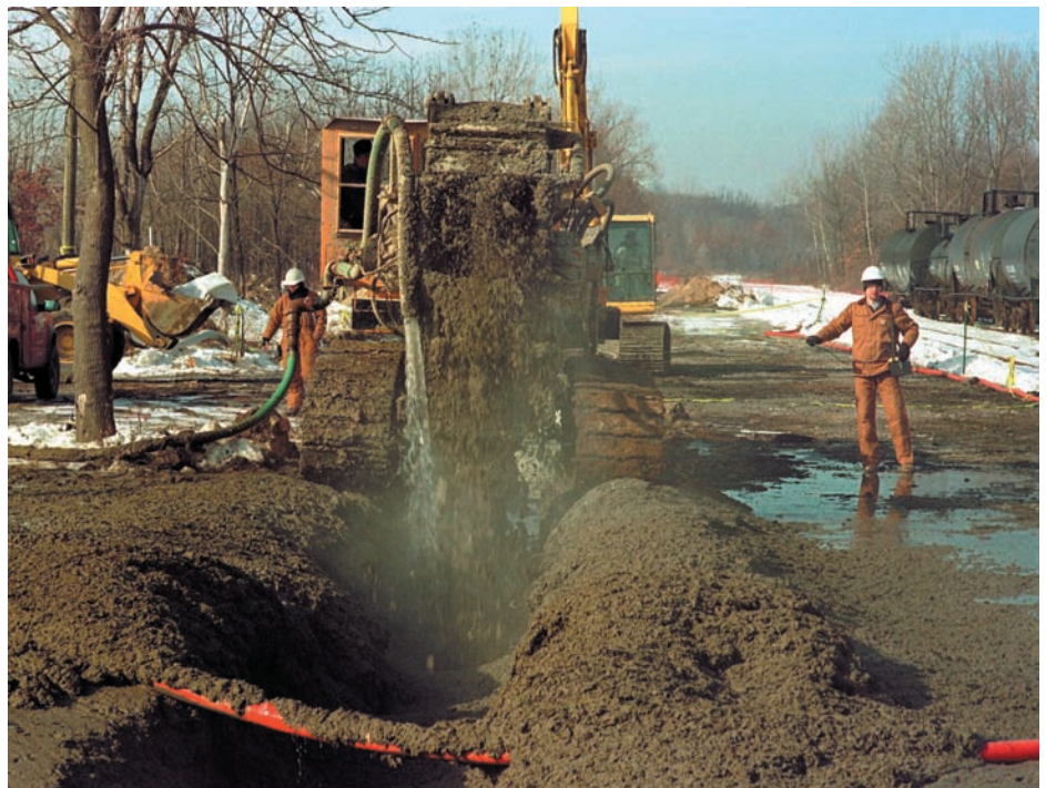
Construction of the separation barrier wall utilizing a trenching machine.
