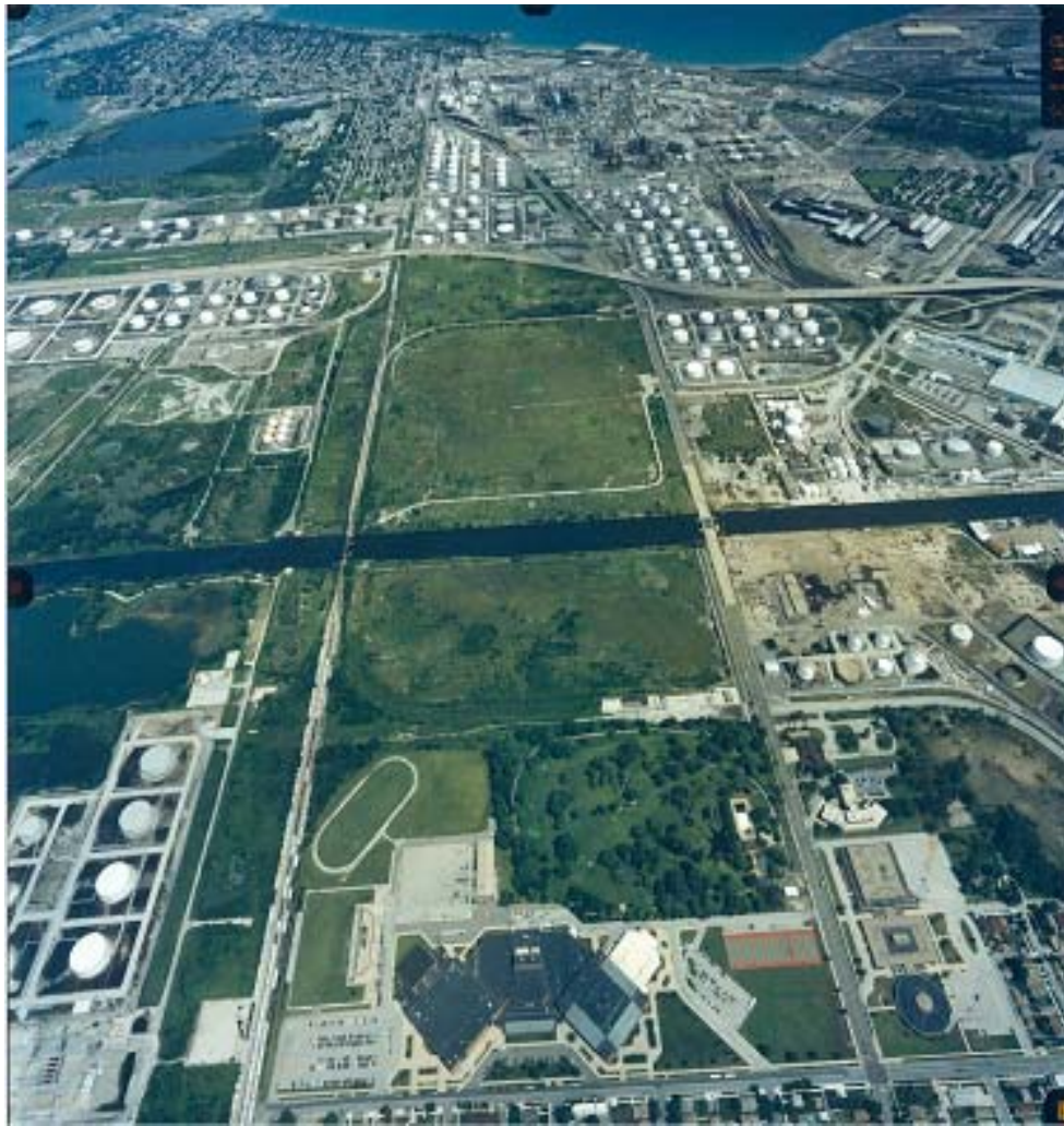
View from the South of the CDF Site (North of Canal) Prior to Construction; Lake Michigan in Background
