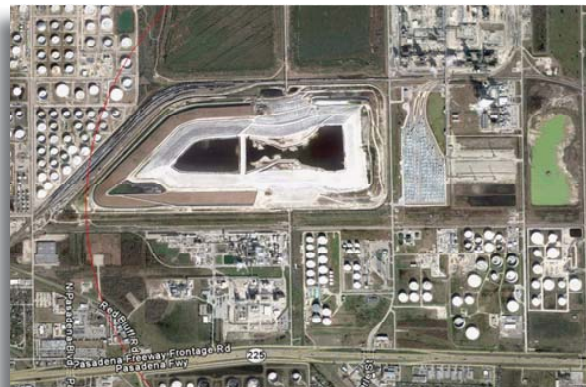
Agrifos, Houston, TX - Gypsum stacks
