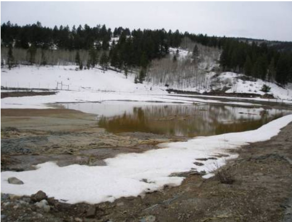
Photo No. 4 – Temporary Cell on CTP. Portion of the geomembrane liner can be seen floating on the surface. View to the west.
