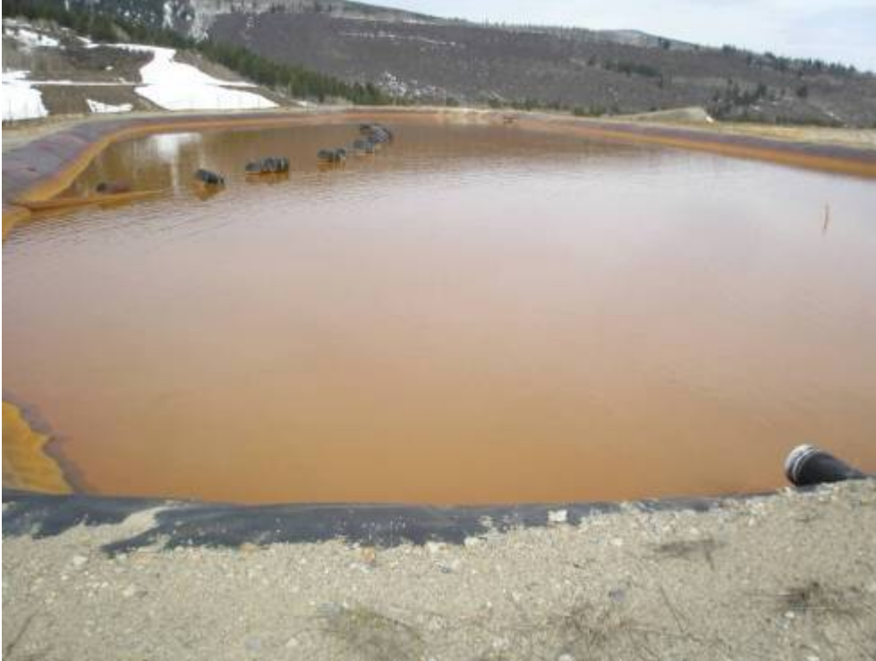
Photo No. 1 – Water Treatment Plant equalization basin. View to west.
