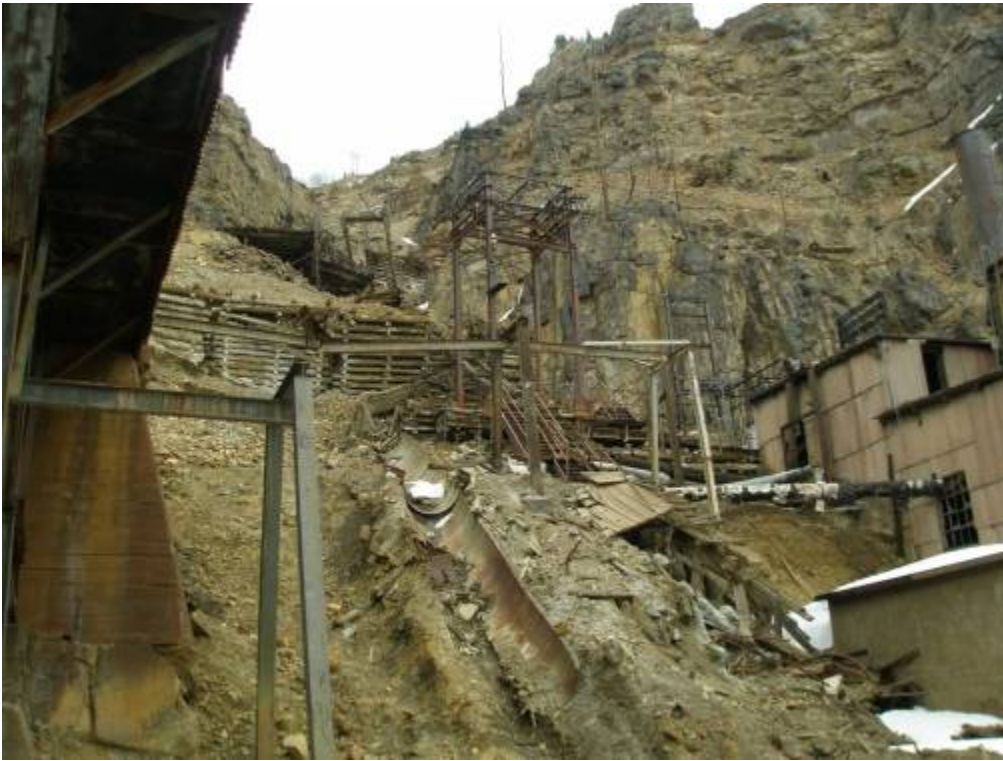
Photo No. 9 – View to east of abandoned mine structures in Belden.
