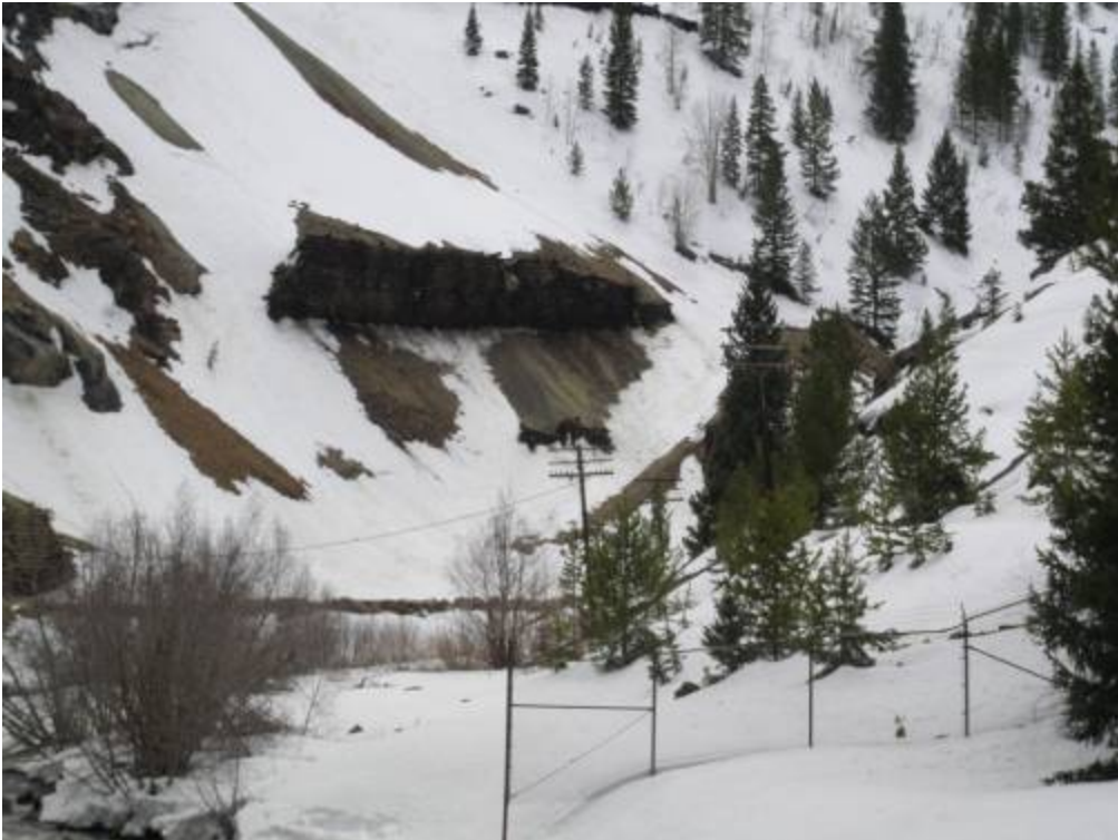
Photo No. 10 – View to south of cribbing near Belden.
