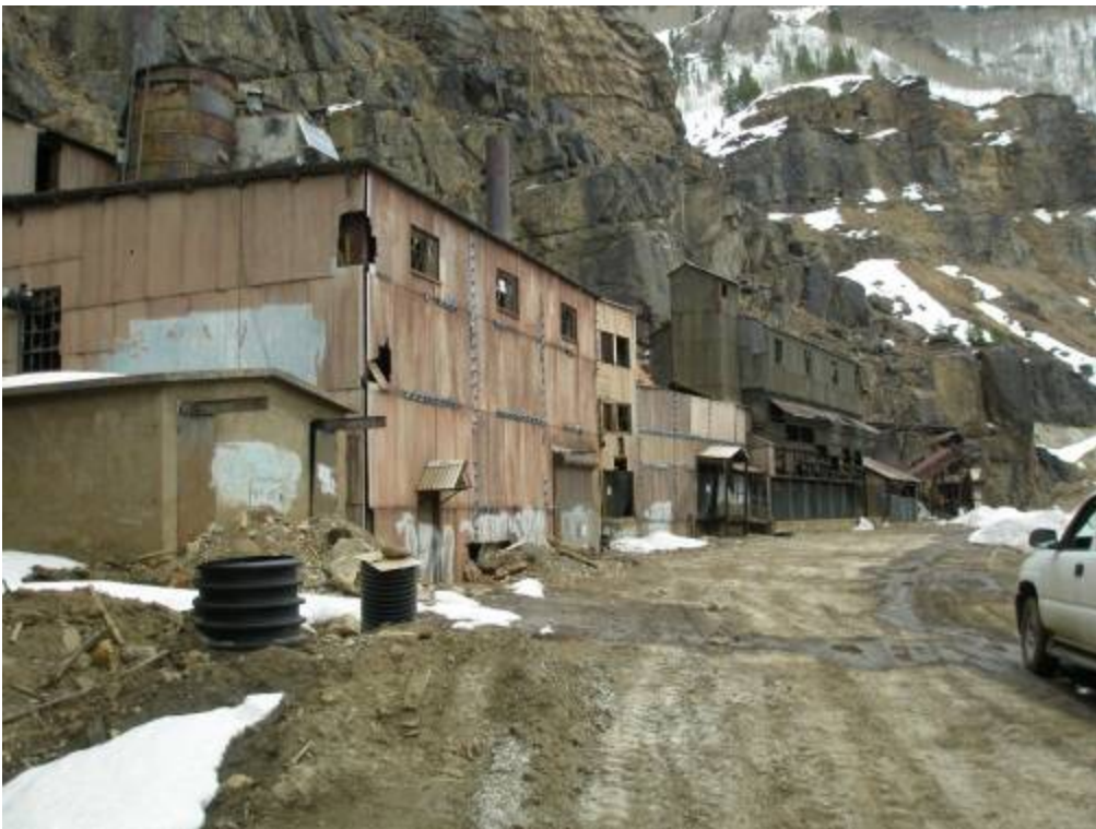
Photo No. 8 – View to South of abandoned mine structures in Belden
