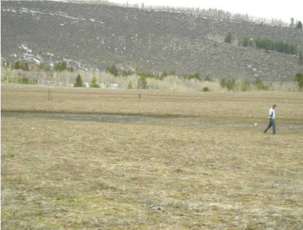
Photo No. 3 – Standing water in area of excessive settlement on southwest portion of CTP. View to west.
