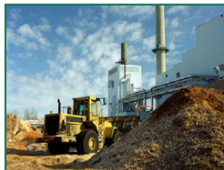
The McNeil Station biopower facility in Burlington, VT
