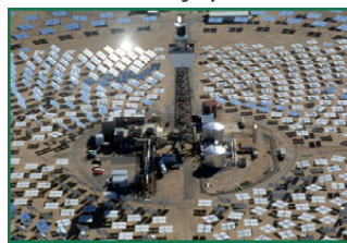
The Solar Two CSP power tower system near Barstow, CA
