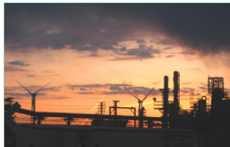
The Steel Winds project in Lackawanna, NY
