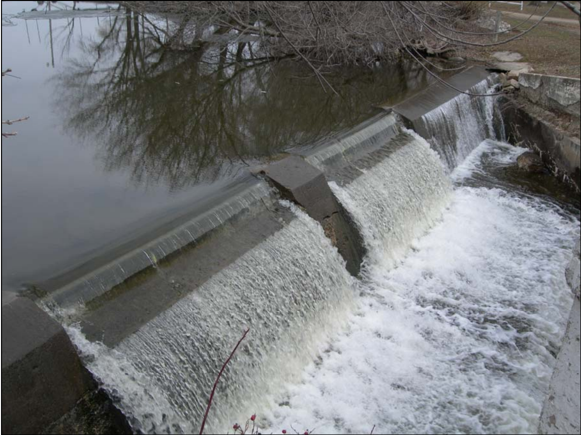
Figure 3. Silver Lake outlet structure to West Branch Little Sioux River.
