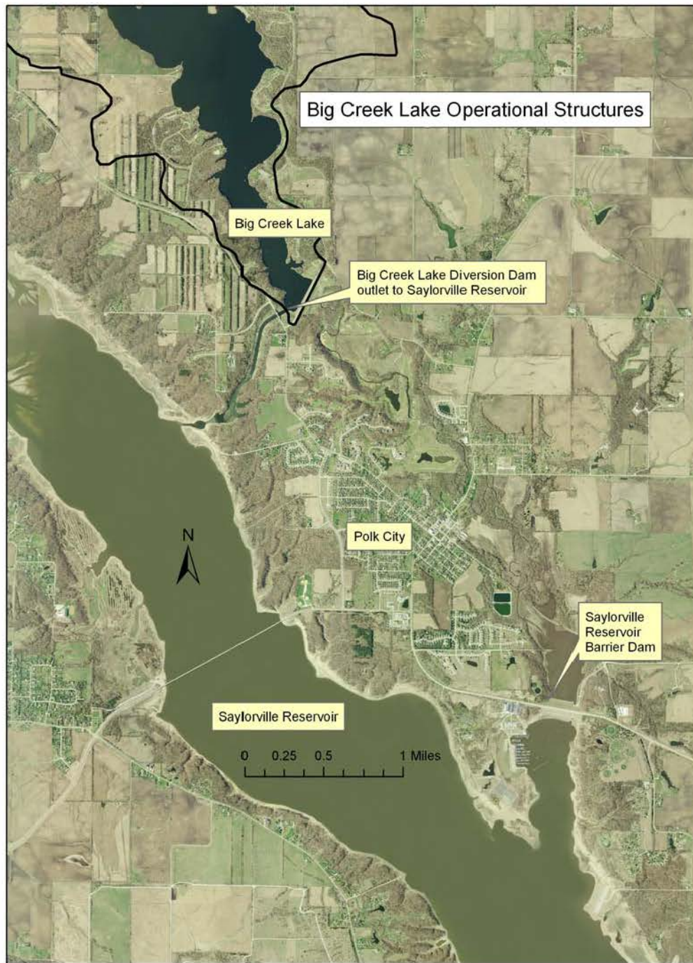
Figure 2-2 Big Creek and Saylorville Lakes Diversion and Barrier Dams
