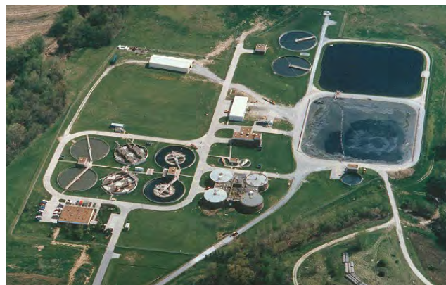
City of Columbia wastewater treatment plant
