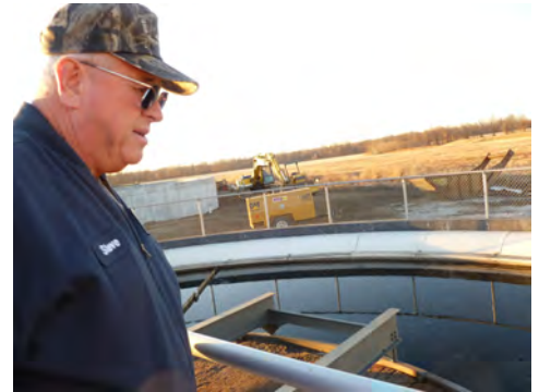
Steve Woodring, Chief Wastewater Operator, overlooks the new clarifier skimmers as part of the 2010-2011 upgrades.
