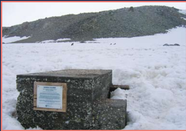
The site of the former British base is marked with concrete foundation blocks.
